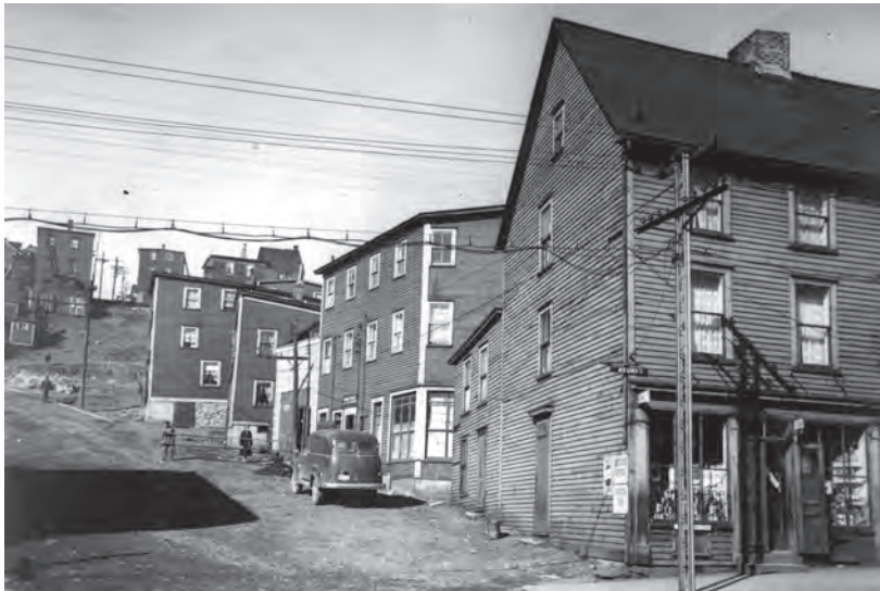
Figure 1.7. Looking up Lime Street from New Gower Street, c. 1950 (CSJA 01-13-014).
